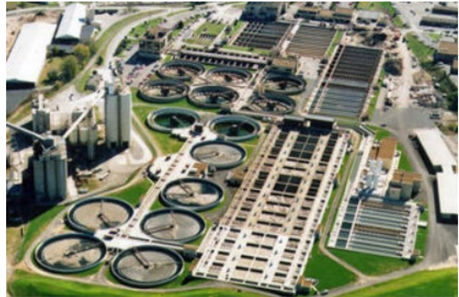
Central Wastewater Treatment Plant, Nashville, Tennessee
